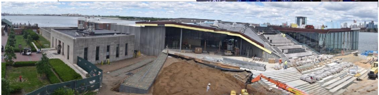
Construction progress of the new Liberty Island museum, June 2018. Ferry pier left side, top. Source: https://libertyellisfoundation.org/statueoflibertymuseum/earthcam.html
